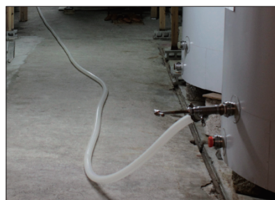
KY SOFT BRAID HOSE Installation Example 2
