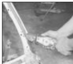
Removing paint and other coating in concave places.
